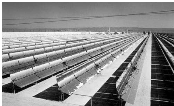
Fig. 1: A Large Solar Mirror Collector Field Located at Kramer Junction, California, USA [2].
